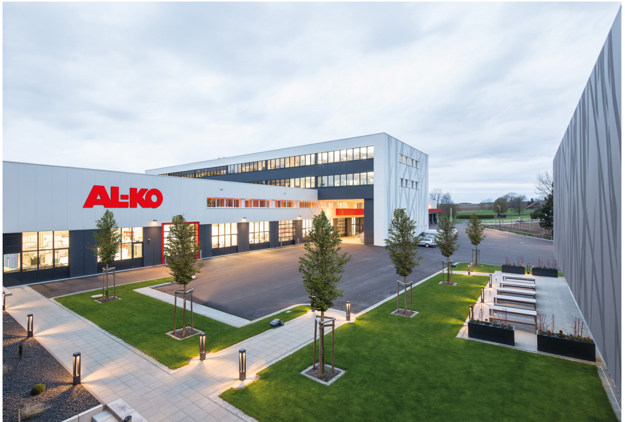
Figure 2: AL-KO Gardentech headquarter in Großkötz [7]
