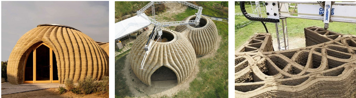
Figure 11: Tecla 3D-printed earth house by WASP (TECLA, 2024)
