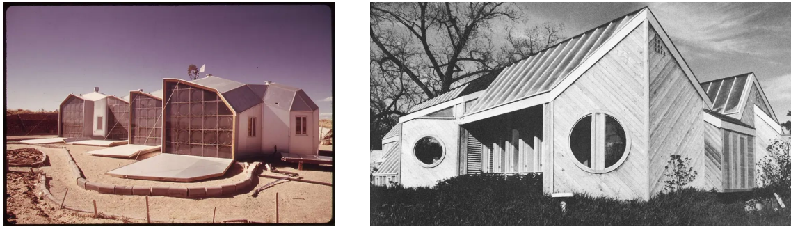
Figure 1: Solar house (1970s) with angled glass for passive heating (Denzer, 2014)
